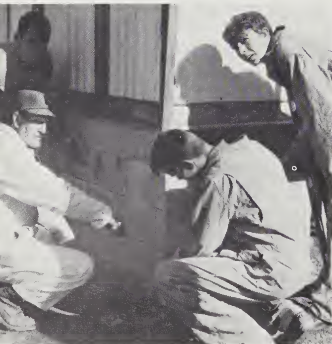
Peeling mortar? Would you believe . . . ?
