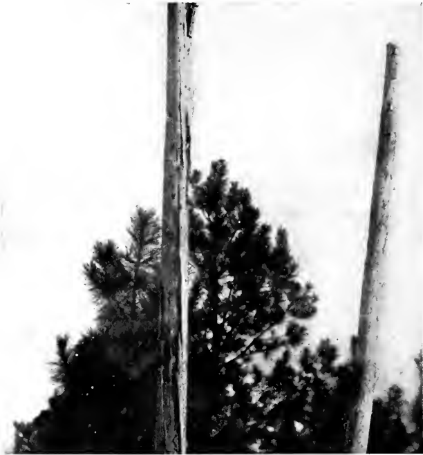
Destruction to a Telegraph Pole caused by Brown-headed Nuthatches
