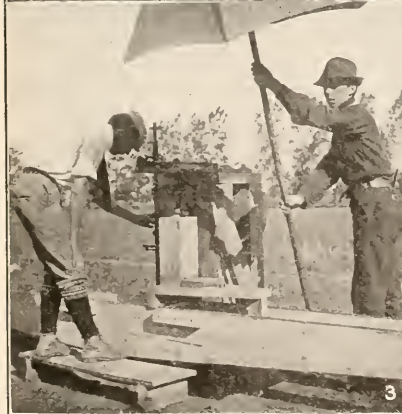
1. Plane Table Work. 2. Lad Signaling Roadman to Move. 3. Reading Microscopically in Precise Measurement Work in the Field. 4. Erecting a Signal Over a Recovered Triangulation Point
