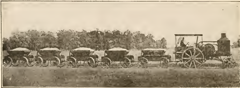
HAULING 22½ YARDS OF CRUSHED ROCK
