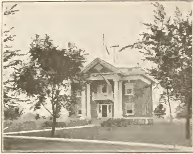
WEATHER BUREAU STATION OF THE "OBSERVATORY" TYPE AT PEORIA
