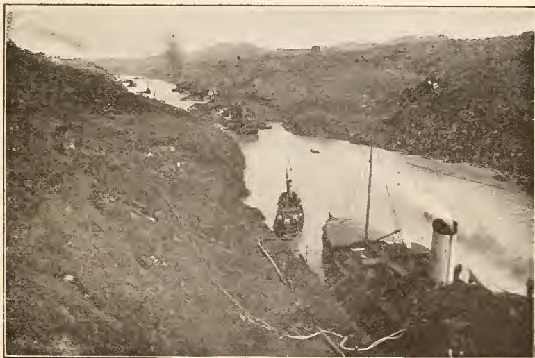
GAILLARD CUT CULEBRA—LOOKING NORTH FROM CONTRACTOR'S HILL, SHOWING BARRIER ACROSS CANAL FORMED BY SLIDES FROM EAST AND WEST BANKS, NOVEMBER 18, 1915
