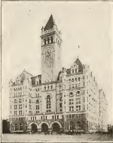
POST OFFICE DEPARTMENT BUILDING
