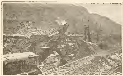
STEAM SHOVELS AT WORK ON THE PANAMA CANAL CULEBRA CUT MAY 20, 1913
