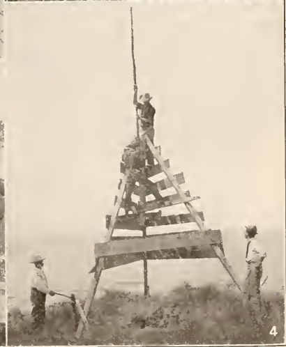
1. Plane Table Work. 2. Lad Signaling Roadman to Move. 3. Reading Microscopically in Precise Measurement Work in the Field. 4. Erecting a Signal Over a Recovered Triangulation Point
