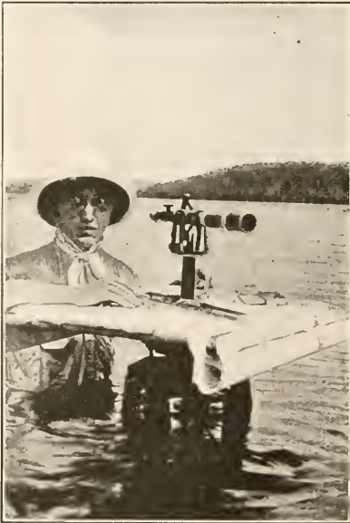
PLANE TABLE WORK IN THE WATER IN THE PHILIPPINES
