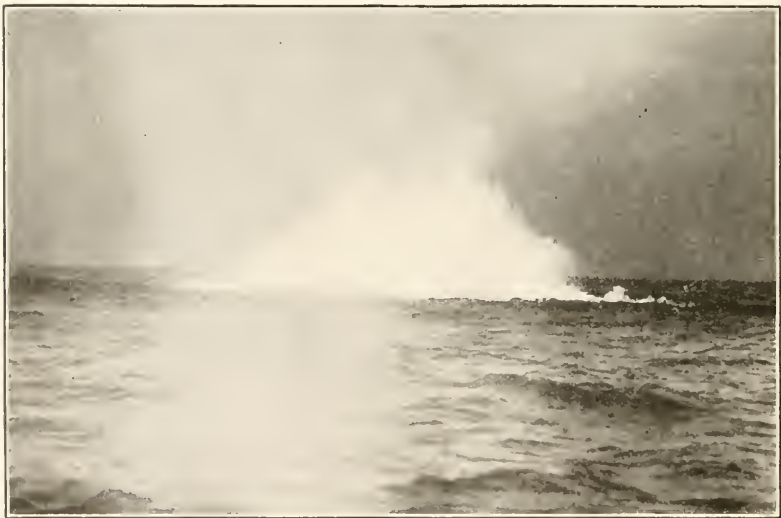
BLOWING UP A SUNKEN MENACE TO NAVIGATION BY MEANS OF SUBMARINE MINES
