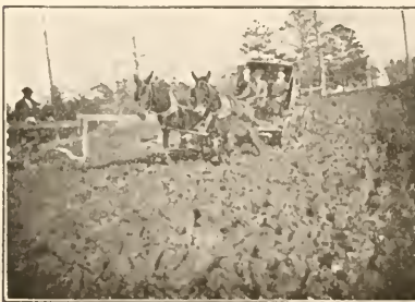
A ROAD BEFORE IMPROVEMENT
