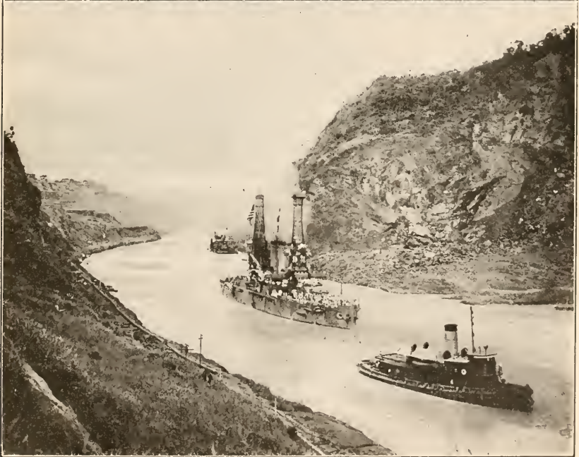
S.S. "CRISTOBAL" IN CULEBRA CUT AT PARAISO ON RETURN TRIP THROUGH CANAL—LOOKING NORTH FROM TOP OF CERRO LUISA, AUGUST 4, 1914 U.S.S. "OHIO" PASSING CUCARACHA SLIDE—LOOKING NORTH, JULY 16, 1915
