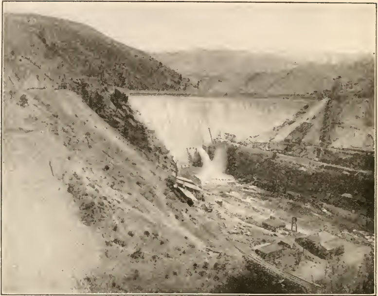
BOISE IRRIGATION PROJECT, IDAHO. HIGHEST DAM IN THE WORLD, 351 FEET FROM BED ROCK TO PARAPET, 1,060 FEET LONG ON TOP
