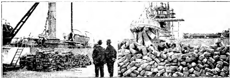
TAKING ON A CARGO OF PIG IRON BY MEANS OF ELECTRIC LIFTING MAGNETS. NOTE HOW THE PIGS FLY TO THE MAGNET
