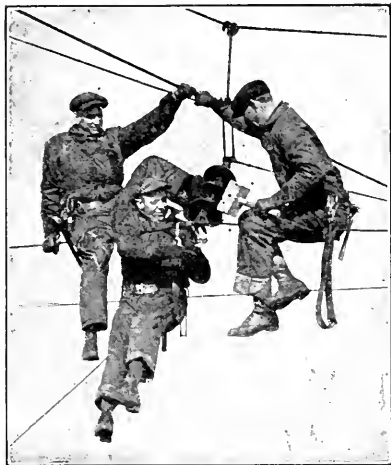
THE HAZARDOUS LIFE OF A RAILROAD LINEMAN
