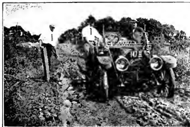
POOR ROAD—TIME IS MONEY—A DELAY
