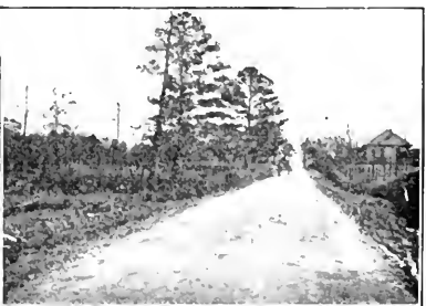
THE SAME ROAD AFTER IMPROVEMENT—CLAY AND GRAVEL CONSTRUCTION
