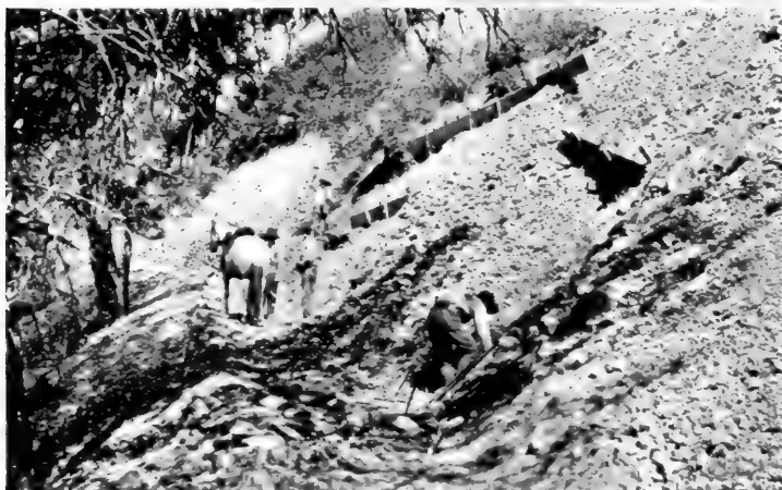
Figure 17. A forest fire lookout station on the top of Lassen Peak, elevation 10,400 feet, Lassen National Forest, California. This cabin was first erected complete in a carpenter's shop in Red Bluff, about 50 miles away. It was then taken to pieces and packed to the foot of Lassen Peak. On the last two miles of its journey it was packed piece by piece on forest officers' backs and finally reassembled on the topmost pinnacle of the mountain. Photo by the author.
