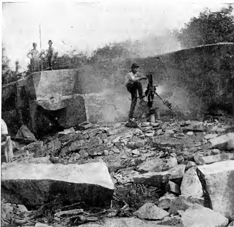
FIG. 57.—A drill operated by compressed air in a quarry
