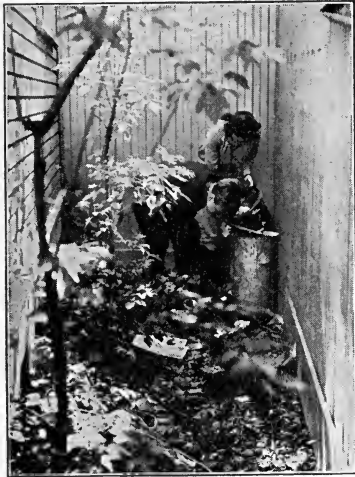
REMOVING A FIRE HAZARD
