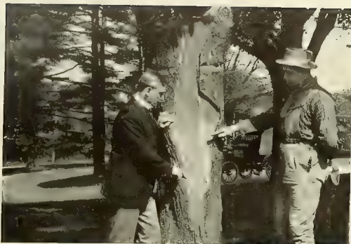
After the Davey treatment. The tree was braced properly, the decayed part removed and the "food" of the tree allowed to reach the roots
