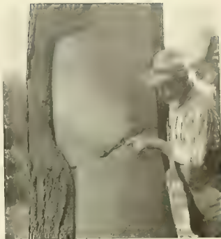
An example of poor cement work done by novices
