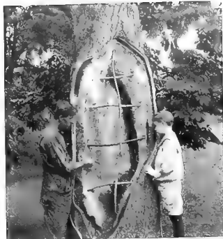
One Davey method of reinforcing cement
