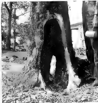
A cavity cleaned out preparatory to filling
