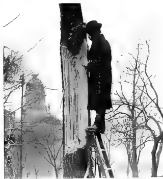
Too long neglected; wind storm split it
