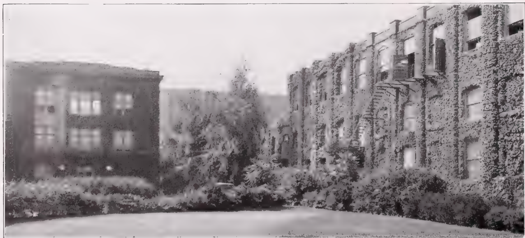
Even the bare walls of factory buildings are suppressed and made beautiful by the thoughtful planting of trees, shrubs and vines. Imagine the scene above without the planting. What a wonderful difference has been created at small cost.
