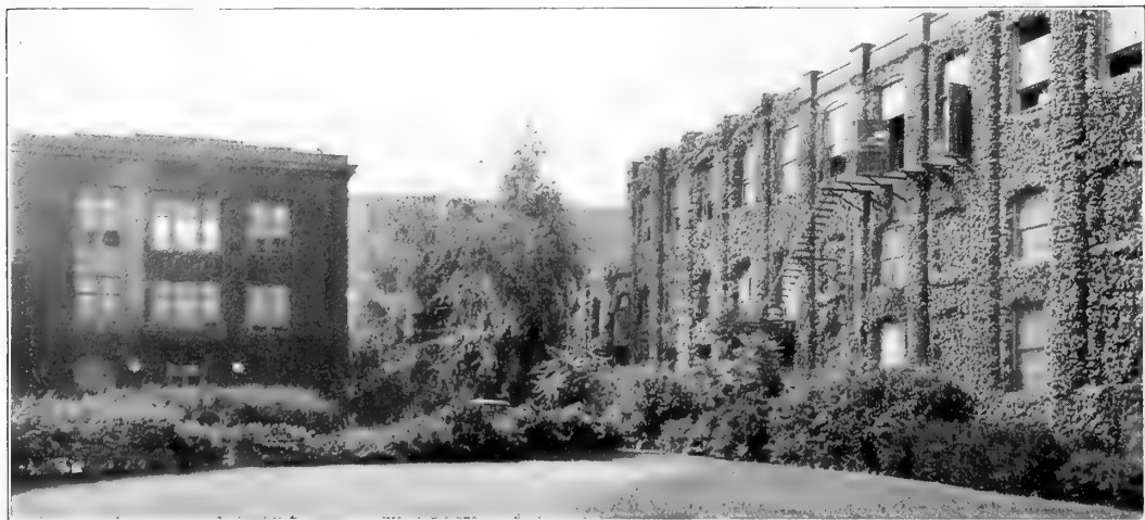
Even the bare walls of factory buildings are suppressed and made beautiful by the thoughtful planting of trees, shrubs and vines. Imagine the scene above without the planting. What a wonderful difference has been created at small cost.
