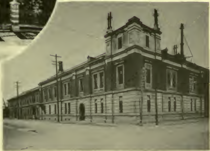
Silk Conditioning House.
