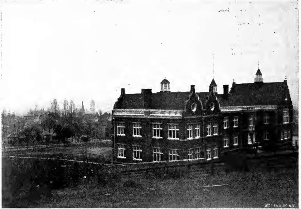
VIEW FROM THE SOUTHWEST.
