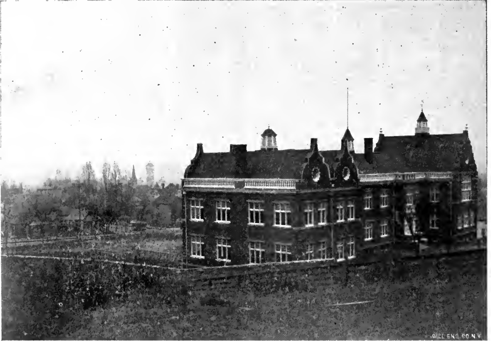
VIEW FROM THE SOUTHWEST.
