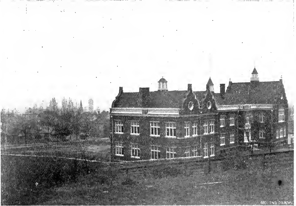
VIEW FROM THE SOUTHWEST.
