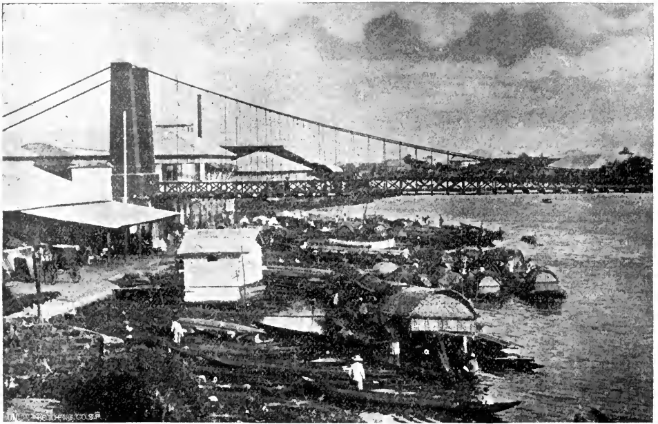
Suspension Bridge across Pasig River, Manila. The picture also shows the large native cascós used as freight lighters on the River and in the Bay.
