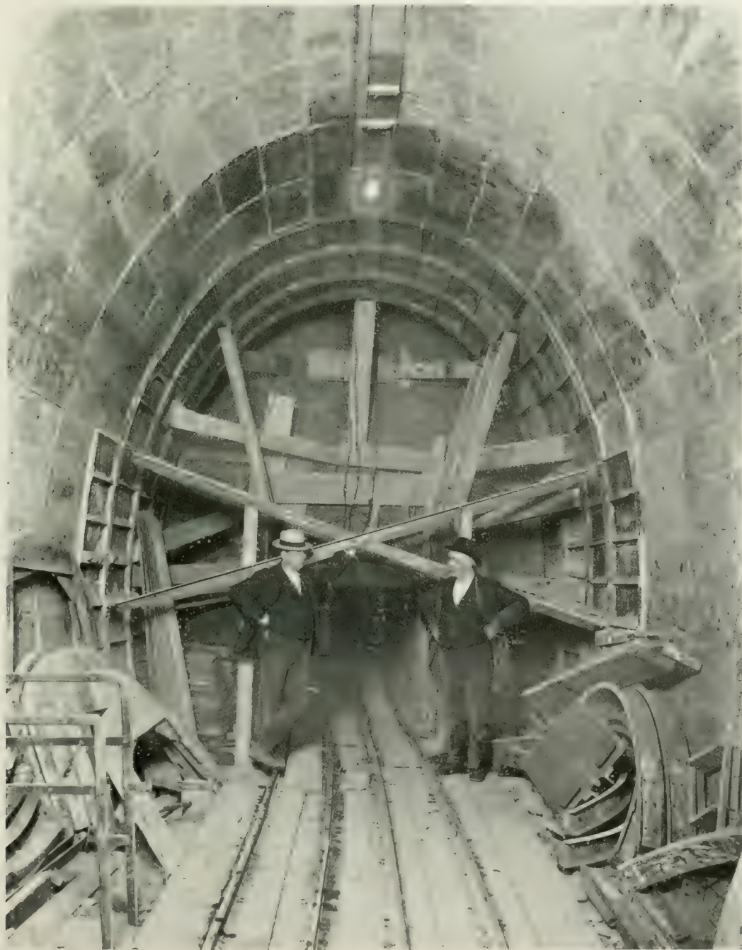
FIG. 5. VIEW OF TRUNK CONDUIT UNDER CONSTRUCTION.
