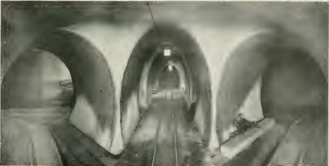
FIG. 11. FOUR-WAY INTERSECTION COMPLETED
