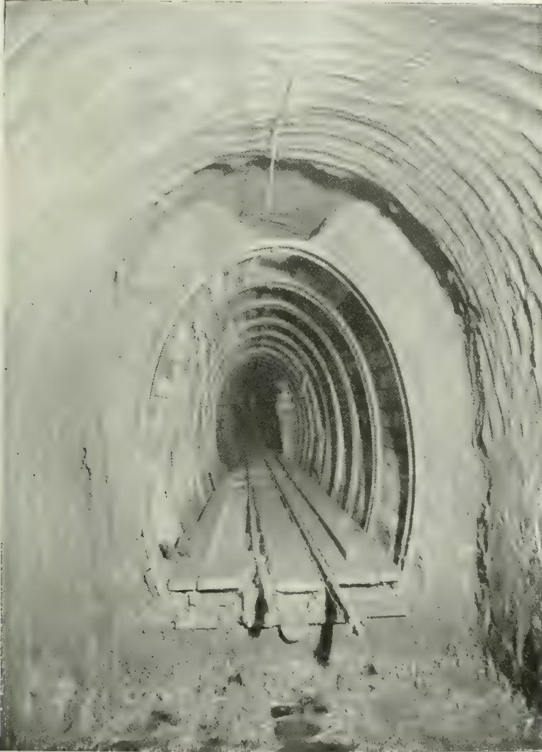
FIG. 4. LATERAL CONDUIT UNDER CONSTRUCTION.
