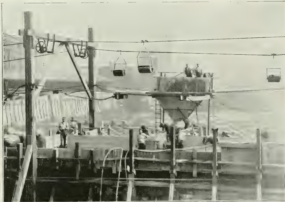
View of a Ropeway recently constructed for the Corporation of Liverpool.
