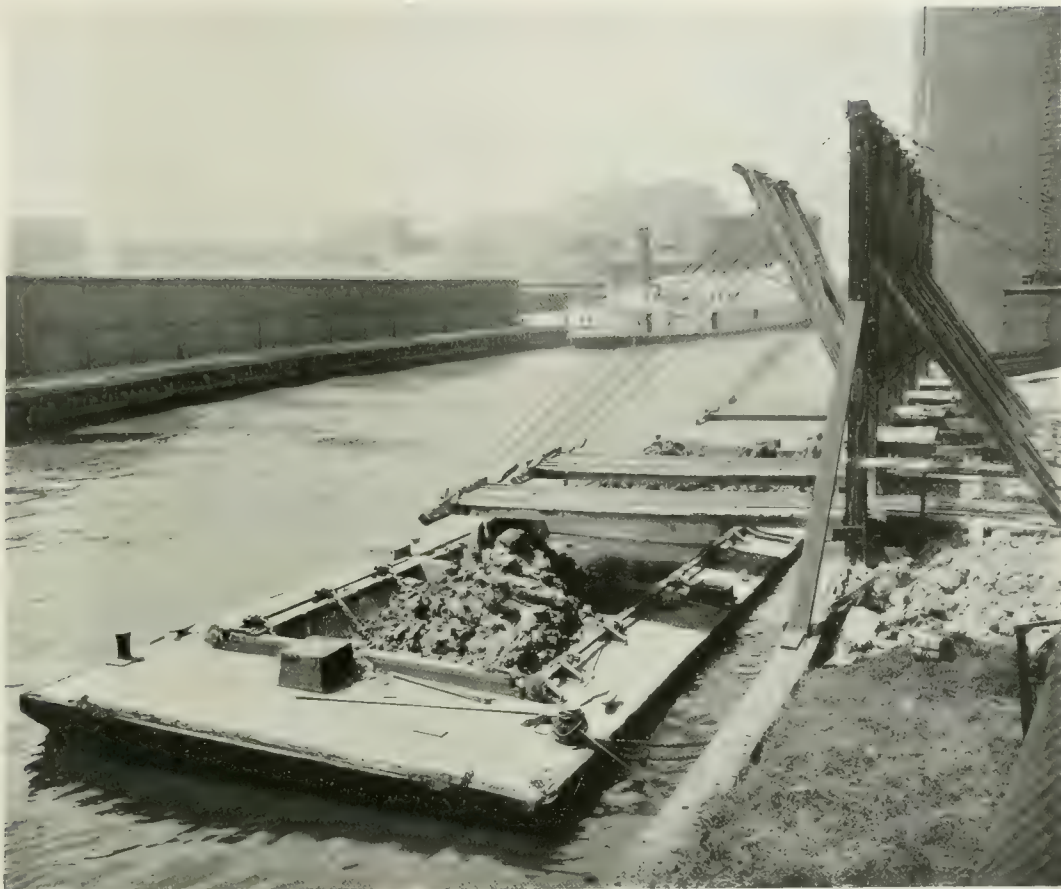
FIG. 10. LOADING SCOWS IN THE RIVER WITH EXCAVATED MATERIAL FROM SHAFT 8.
