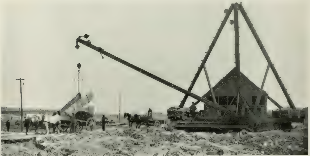
FIG. 7 UNLOADING THE ENCAVATED CLAY AT THE LAKE FRONT. Lifting away the side boards of the wagon bed.
