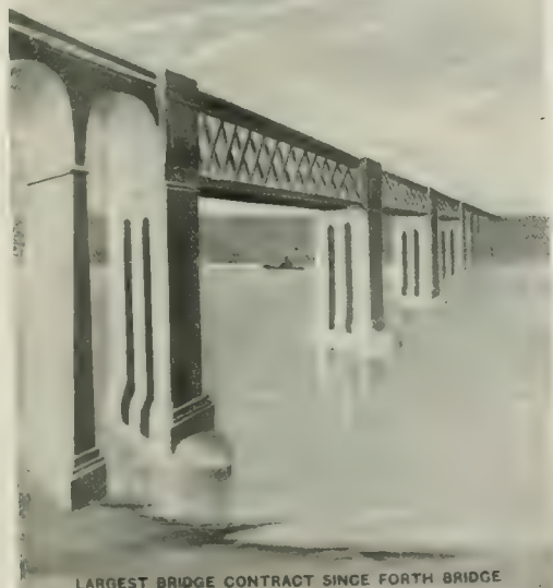
LARGEST BRIDGE CONTRACT SINCE FORTH BRIDGE
