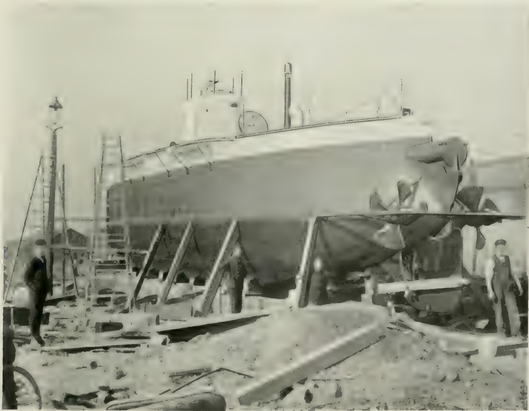
THE SUBMARINE TORPEDO-BOAT "PROTECTOR" ON THE STOCKS, SHOWING SIDE RUDDERS AND TWIN SCREWS.
