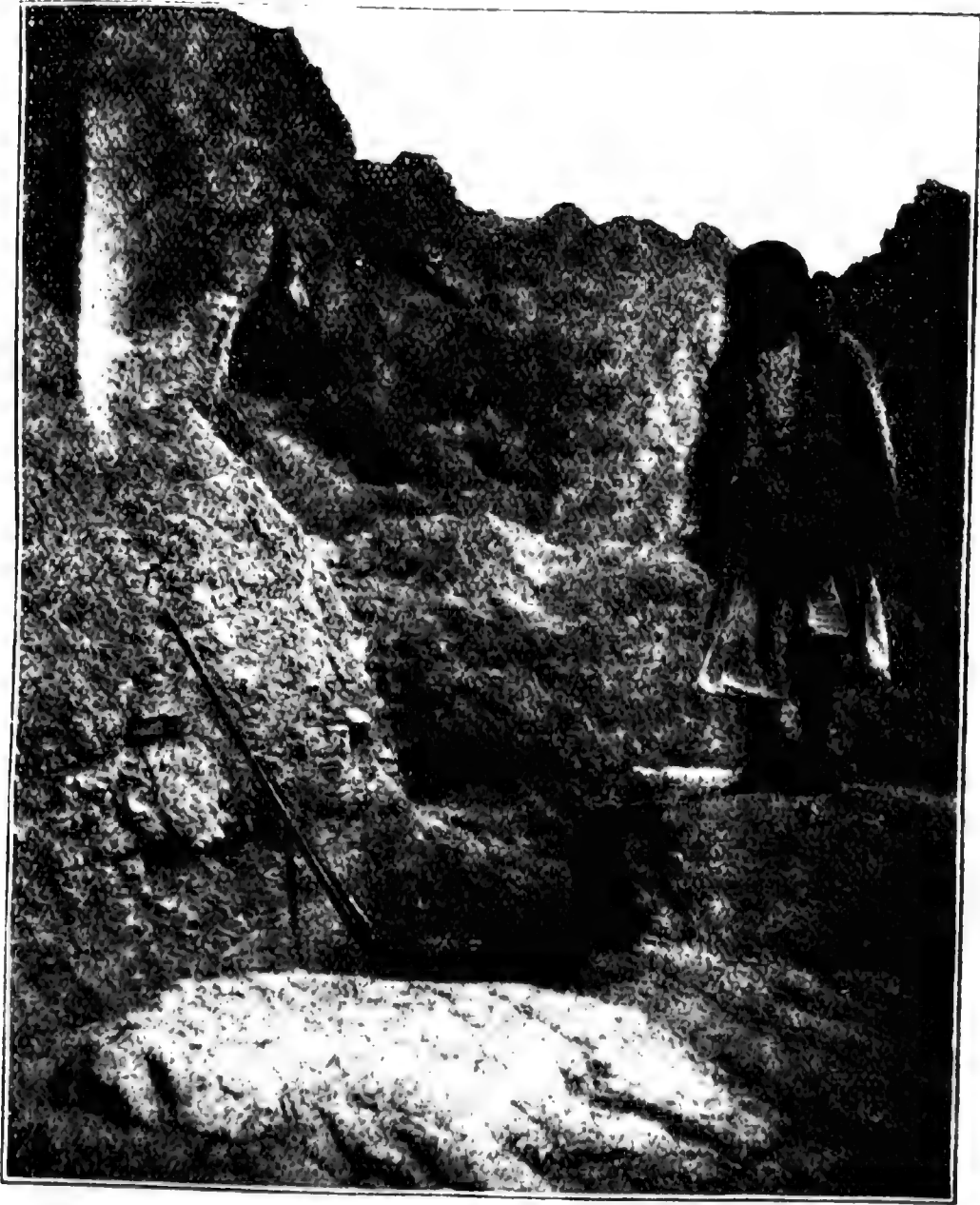
FIG. 2.—Open rock-cut Aqueduct in Wâdy Kumerân, near the beginning. Gun is placed in the channel.
