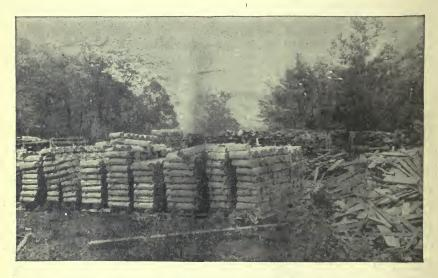
Fig. 18. Mop handle and chair dowels and mill waste from which they are manufactured.
