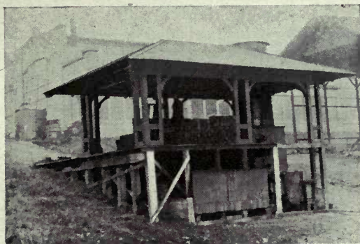
WOOD DISTILLATION PLANT
