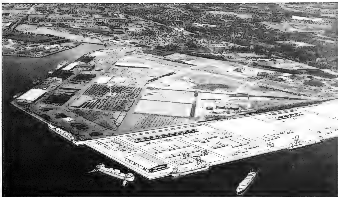
Figure 5. A modern container terminal is being constructed at an abandoned airport in Baltimore harbor. Modern port development may free large areas of obsolete port facilities for other public uses. (Port of Baltimore photo)
