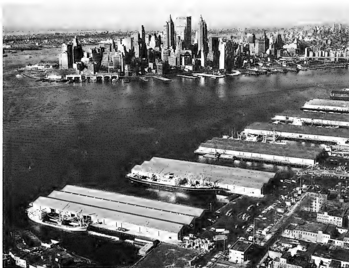
Figure 1. Virtually every population and industrial center is also a major port. (Port of New York Authority photo)
