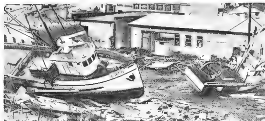
Figure 2. General view of Kodiak, Alaska, showing damage caused by sea-wave resulting from earthquake, March 28, 1964. (ESSA photo)
