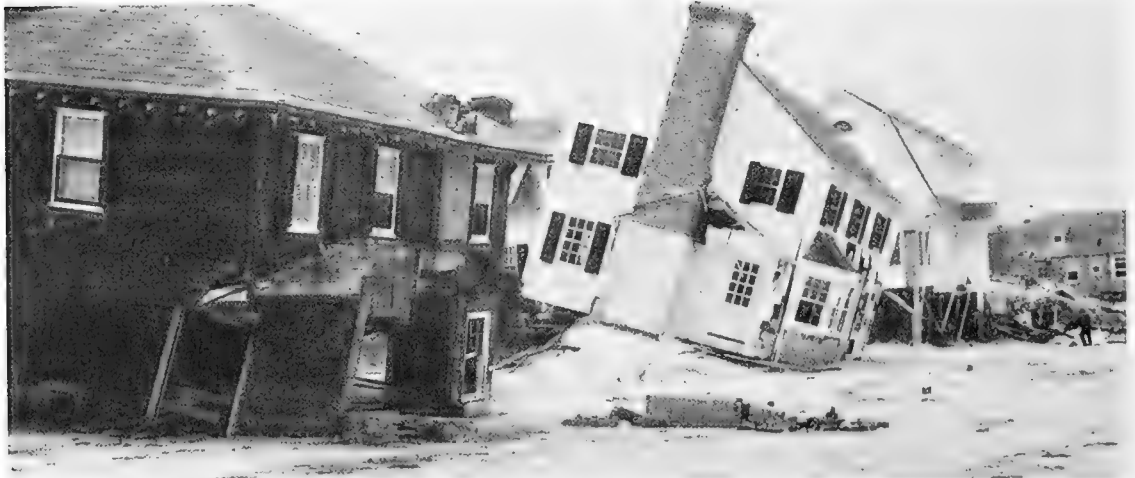
Figure 5. Storm damage of Virginia Beach indicates there may be inadequate controls in the protection and development of coast lands.
