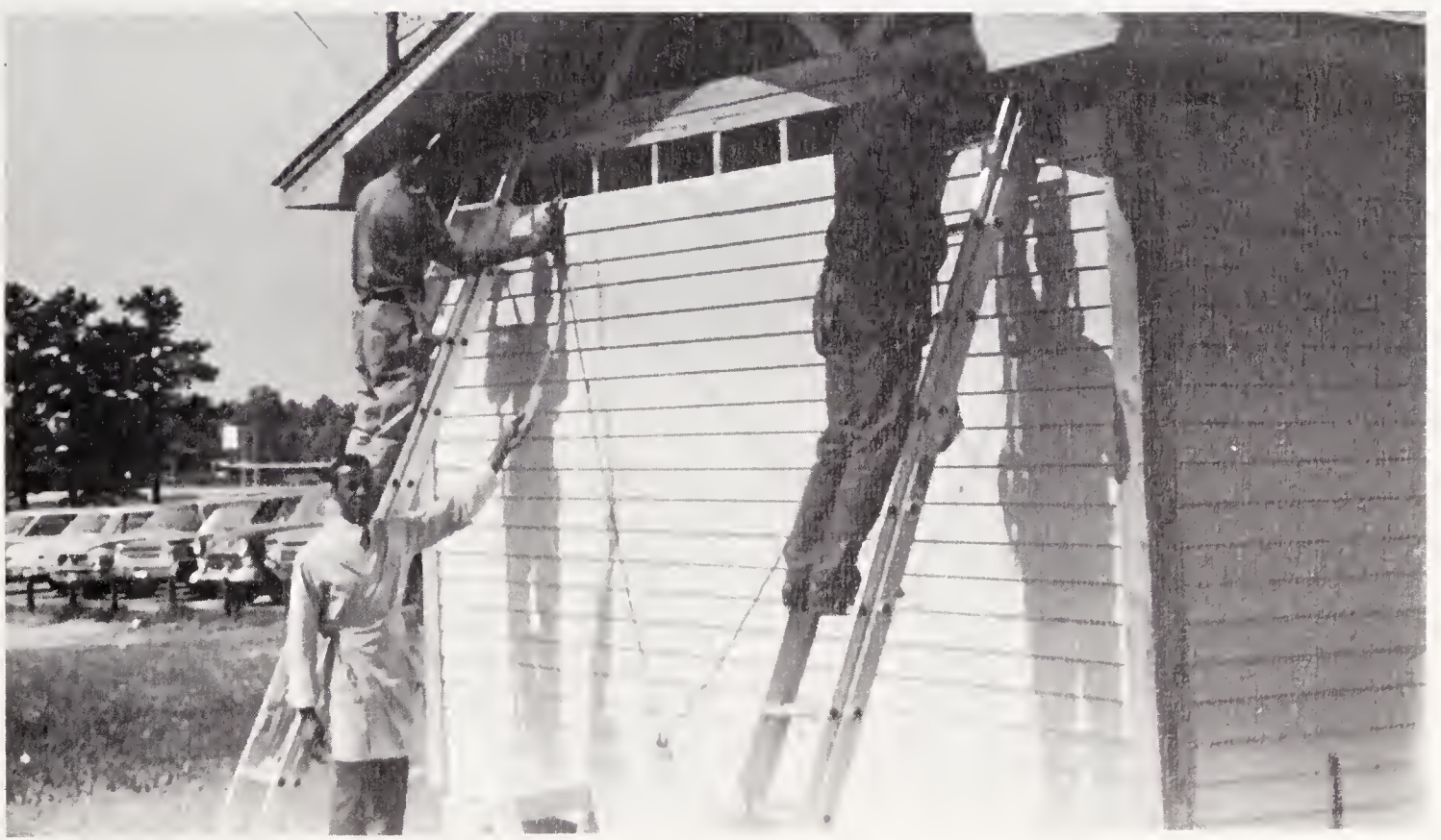
Finishing touch being applied to "school" house.
