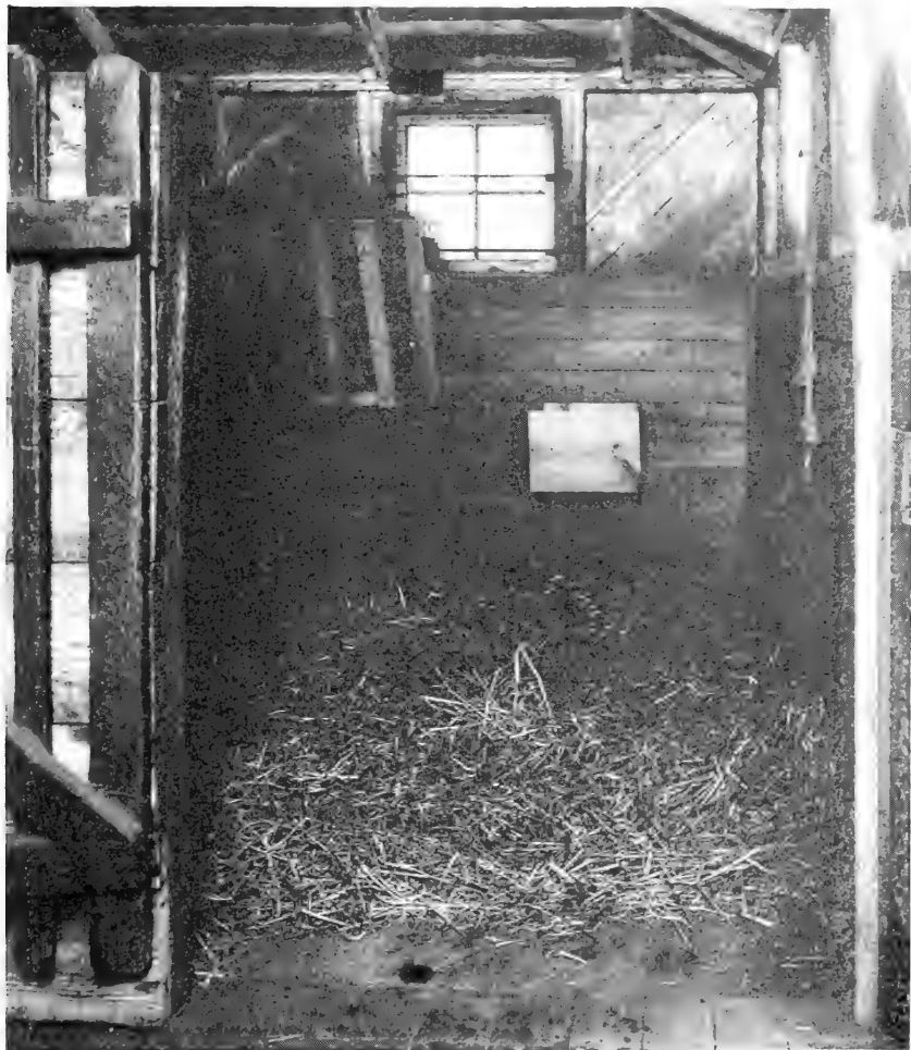
Figure 11.—Type of sanitary box stall. Note feed box and hayrack raised above the ground.
