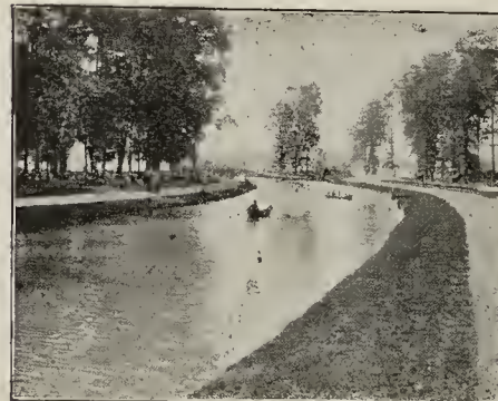
LOOP CANAL, LOOKING NORTHERLY
