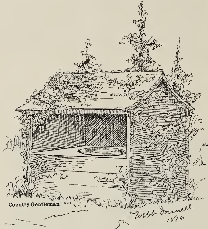
ROAD SIDE SHELTER HOUSE FOR WATERING TROUGH.
