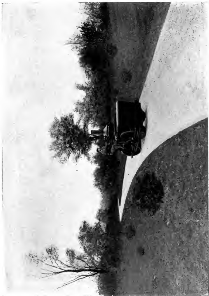
FIG. 16.—Park Walk. Drainage in Grass Gutters. Rolling being Done by Special Tandem Roller. 49
