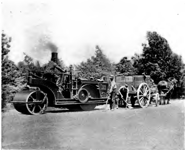
Courtesy Buffalo Steam Roller Co. FIG. 38.—Pavement Repairs at Boston. 121
