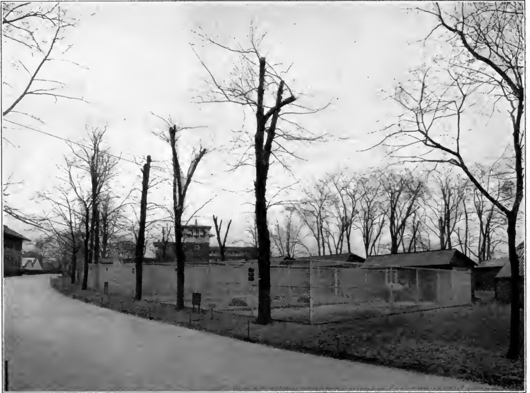
PLATE No. 364. FENCE CONSTRUCTION
