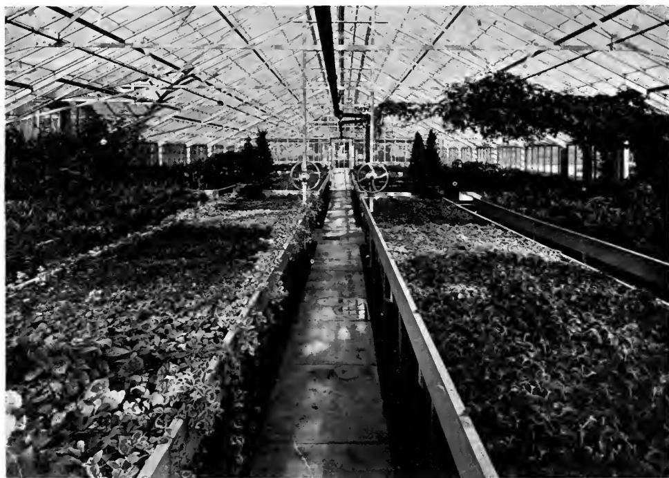
PLATE No. 253. IRON FRAME CONSTRUCTED HOUSE
