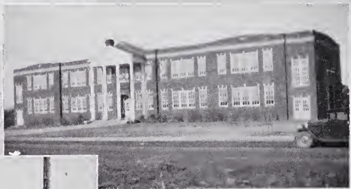
ELEMENTARY SCHOOL BLDG.
