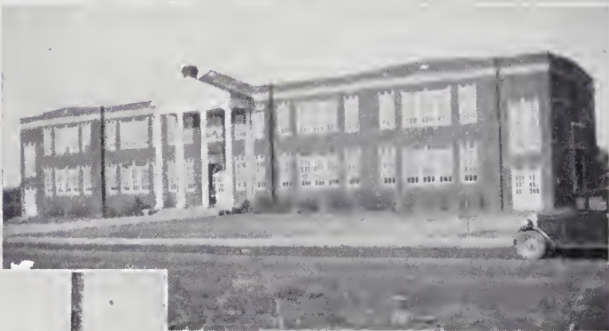
ELEMENTARY SCHOOL BLDG.
