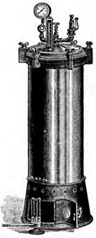
Fig. 40.—Modern autoclave.
