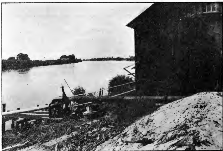
FIG. 128. Centrifugal pump and discharge pipe which carries water from the Sacramento River over a levee into a pear orchard.
