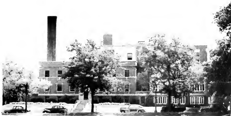
PEKIN PUBLIC HOSPITAL built in 1913 enlarged in 1931 and 1940
