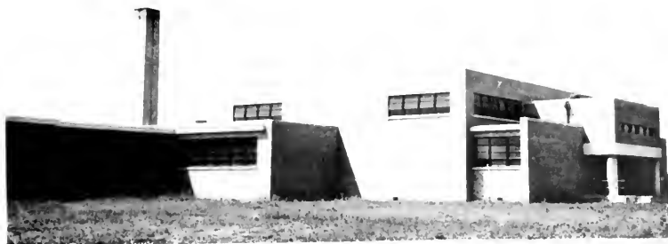
THE NEW FEARN WILSON SCHOOL completed in 1940.
