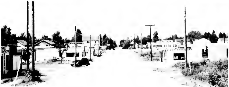
New Business Section on Derby Street
