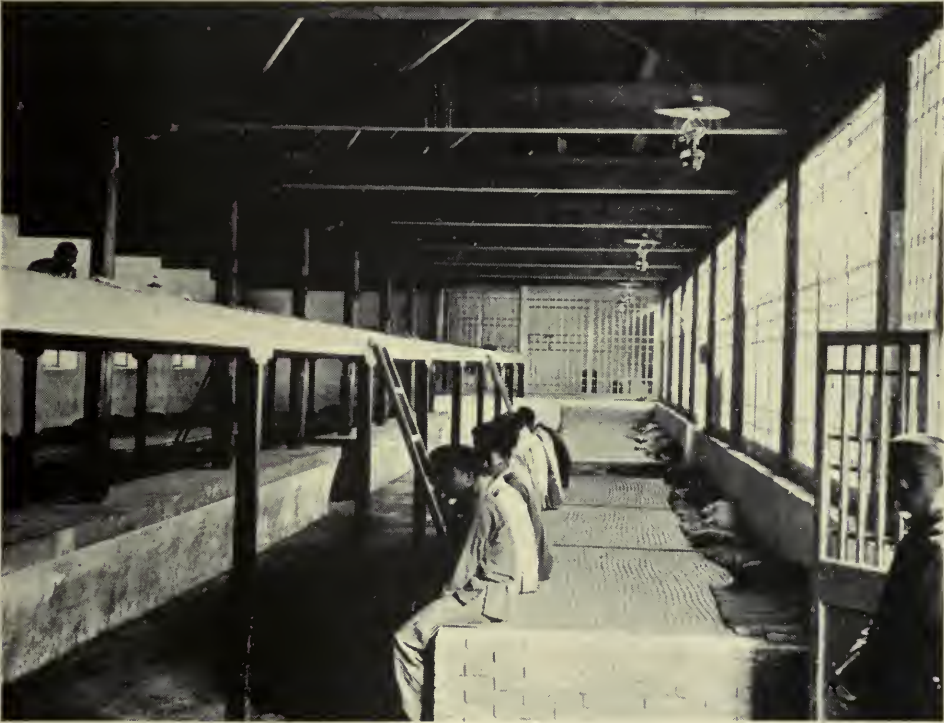
REFORM SCHOOL DORMITORY.
