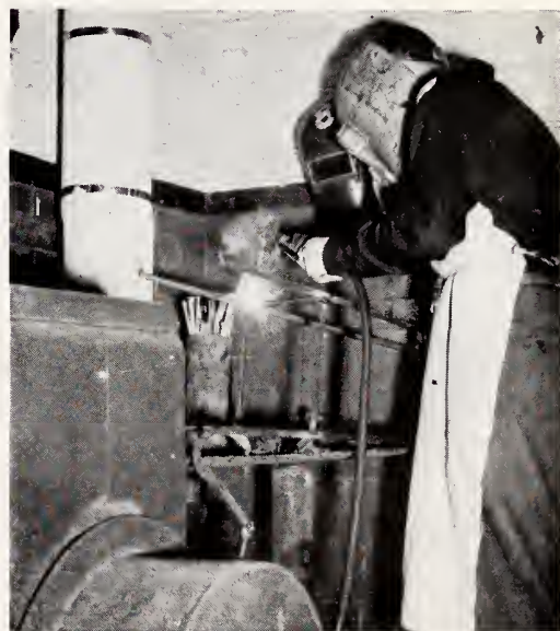
Electric welding mends our time and our equipment.
