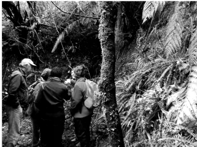
Embankment behind the old toilet block at Cement Creek – Photo: Lee Denis
