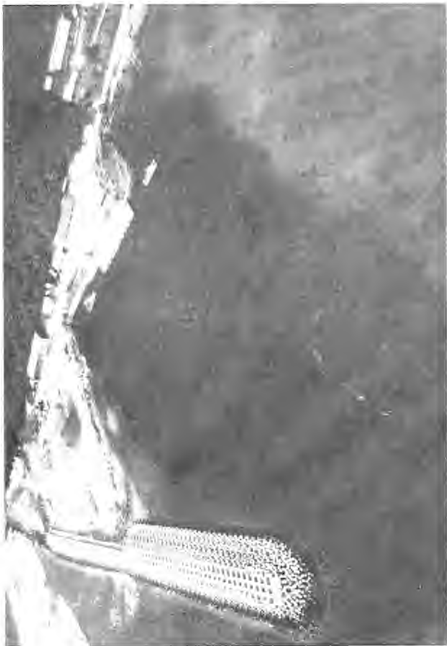
Figure 10. Aerial photograph of Ofu Harbor breakwater (1996)
