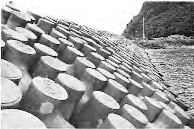
Figure 5. Tribar armor units used on Ofu Harbor breakwater
