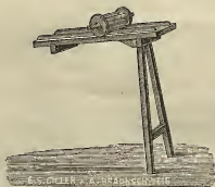
Fig. 3.— Mechanical Butter-worker suitable for small Dairies.
