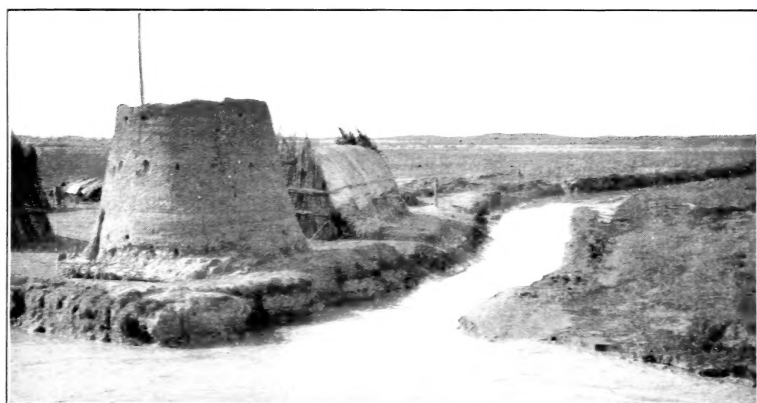
FIG. 3.—INTAKE OF IRRIGATION CANAL ABOVE BASSORAH.
