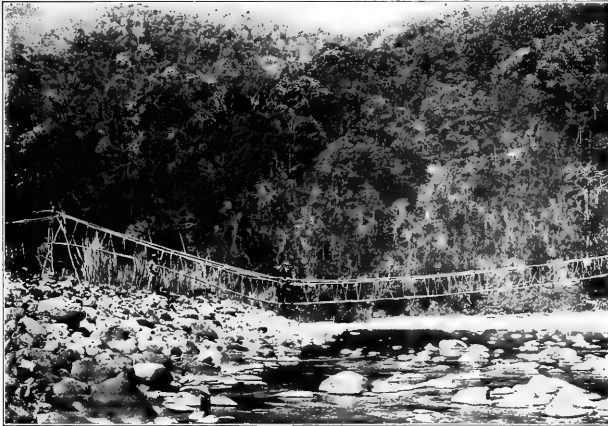
Fig. 2. Rattan bridge built by Mangyans, near Sablayan.
