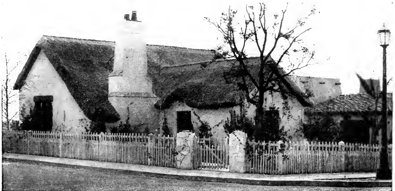
When Fox welcomed John McCormack to Movietone City, they built him this bit of old Ireland to make him feel at home. Every bit of thatch in the roof had to be fireproofed—not an old Irish custom
