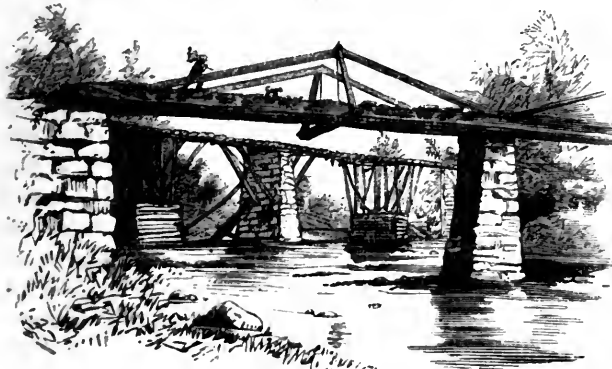
Bridge Across Platte Creek
