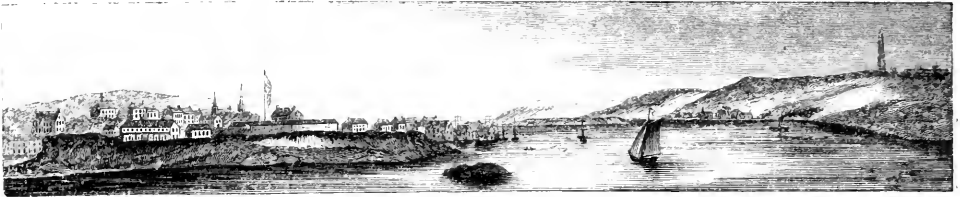
NEW LONDON HARBOR, LOOKING NORTH. 2
