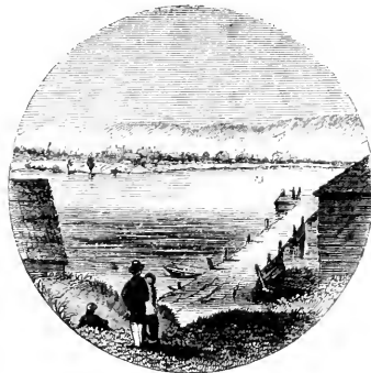
CHIMNEY POINT LANDING. 3
