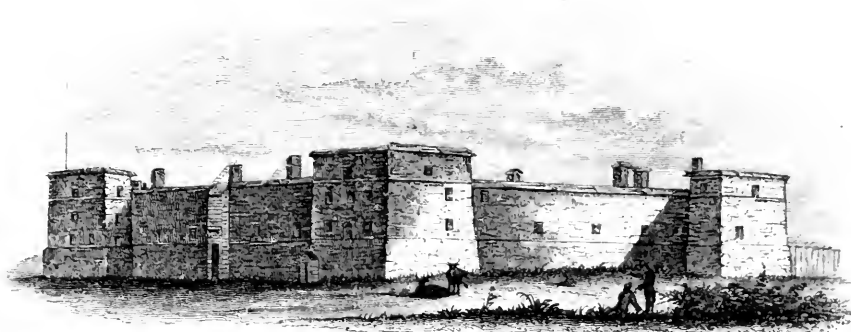
FORT AT CHAMBLY. 1
