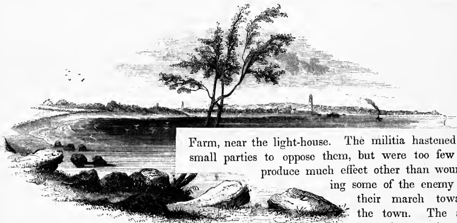
VIEW OF THE LANDING-PLACE OF ARNOLD. 2
