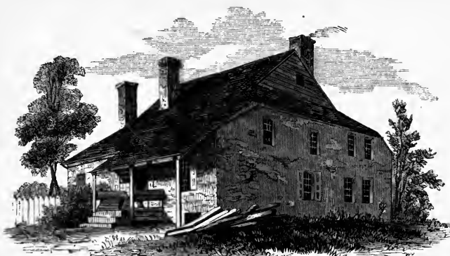
WASHINGTON'S HEAD-QUARTERS AT NEWBURGH. 1
