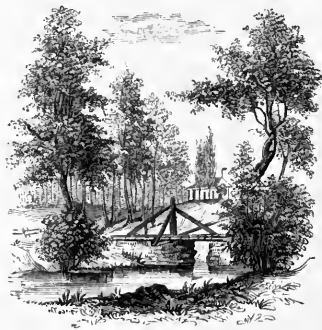
BRIDGE OVER SLEEPY HOLLOW CREEK.
