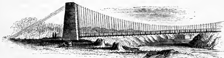
PART OF NIAGARA SUSPENSION BRIDGE. 2
