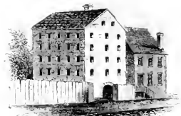
SUGAR-HOUSE IN LIBERTY STREET.*
