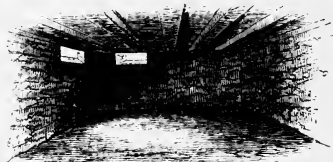
CELLAR OF THE REIDSEL HOUSE.
