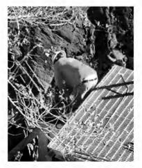
to enhance access to spawning areas for endangered spring-run Chinook salmon. The contractor was pouring the last few walls connecting the zig-zagging metal-caged fish ladder to the hole in the rock face were the old fish ladder had been. Construction started in 2016, but the ladder had to be redesigned when the cliffside that it was to be built on slid into the creek.
