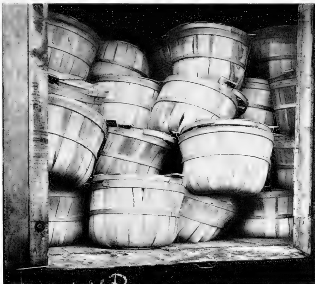
Fig. 27. Faulty methods in stowing lead to this sort of damage.
