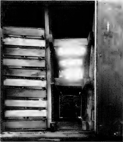
Fig. 96. A pair of gates in place showing ease with which efficient bracing is accomplished.
