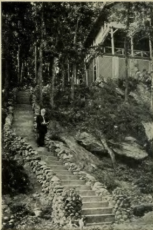
Fig. 12. Example of deficient footing for the house, and of incongruous steps
