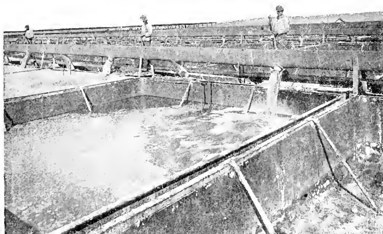
Crystallizing Pans—Full, Filling, and Empty.
