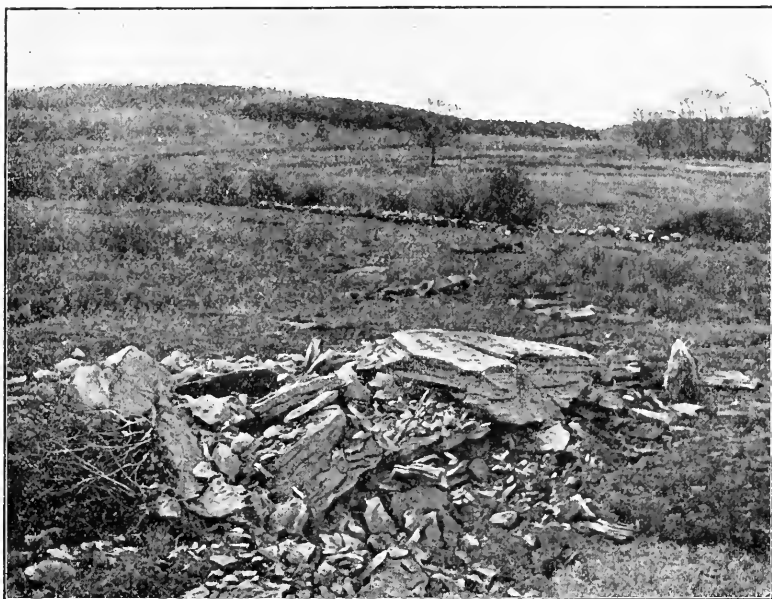
Same Rock Shattered by the Explosion of Dynamite.
