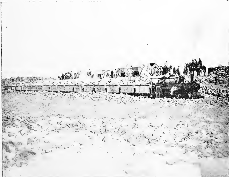
Loading Caliche into Railway Trucks.
