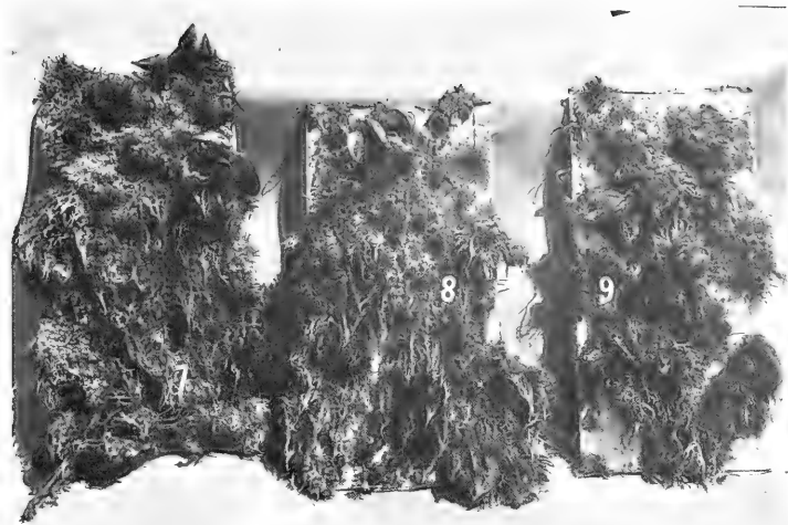
Figure 5. Biological growth over painted carbon steel panels.
