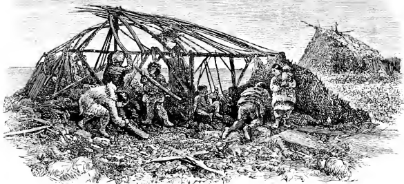
FRAME-WORK OF TCHUKTCHI HOUSE.
