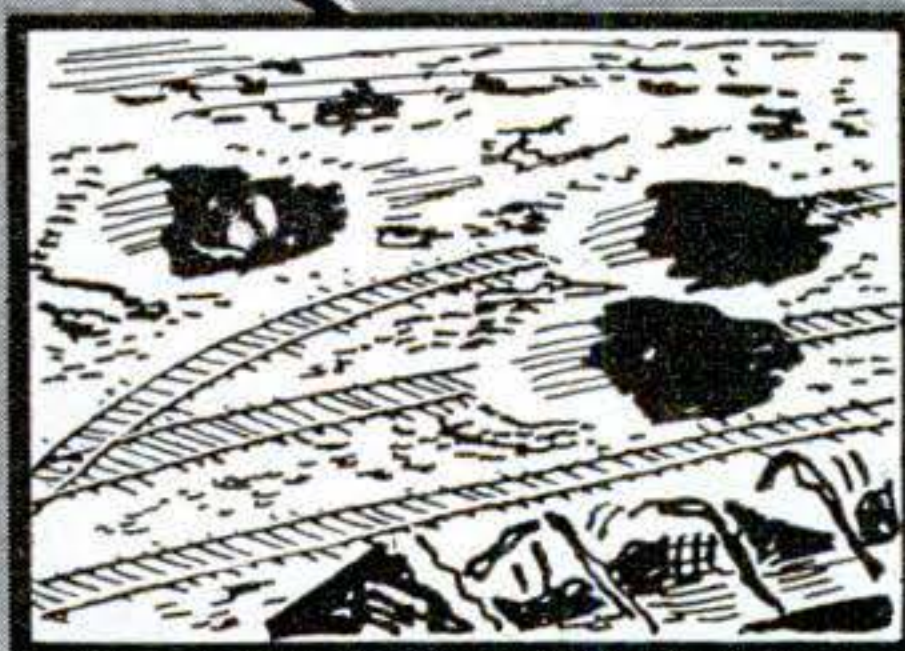
RAILROAD YARDS are now a mass of twisted rails, smashed switches. Repairs will be slow
