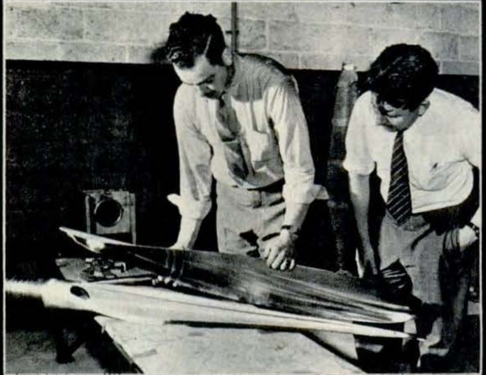
2 When specifications have been met, the camber, or pushing side of the blade, is fitted to the shaped forging to form the completed hollow unit
