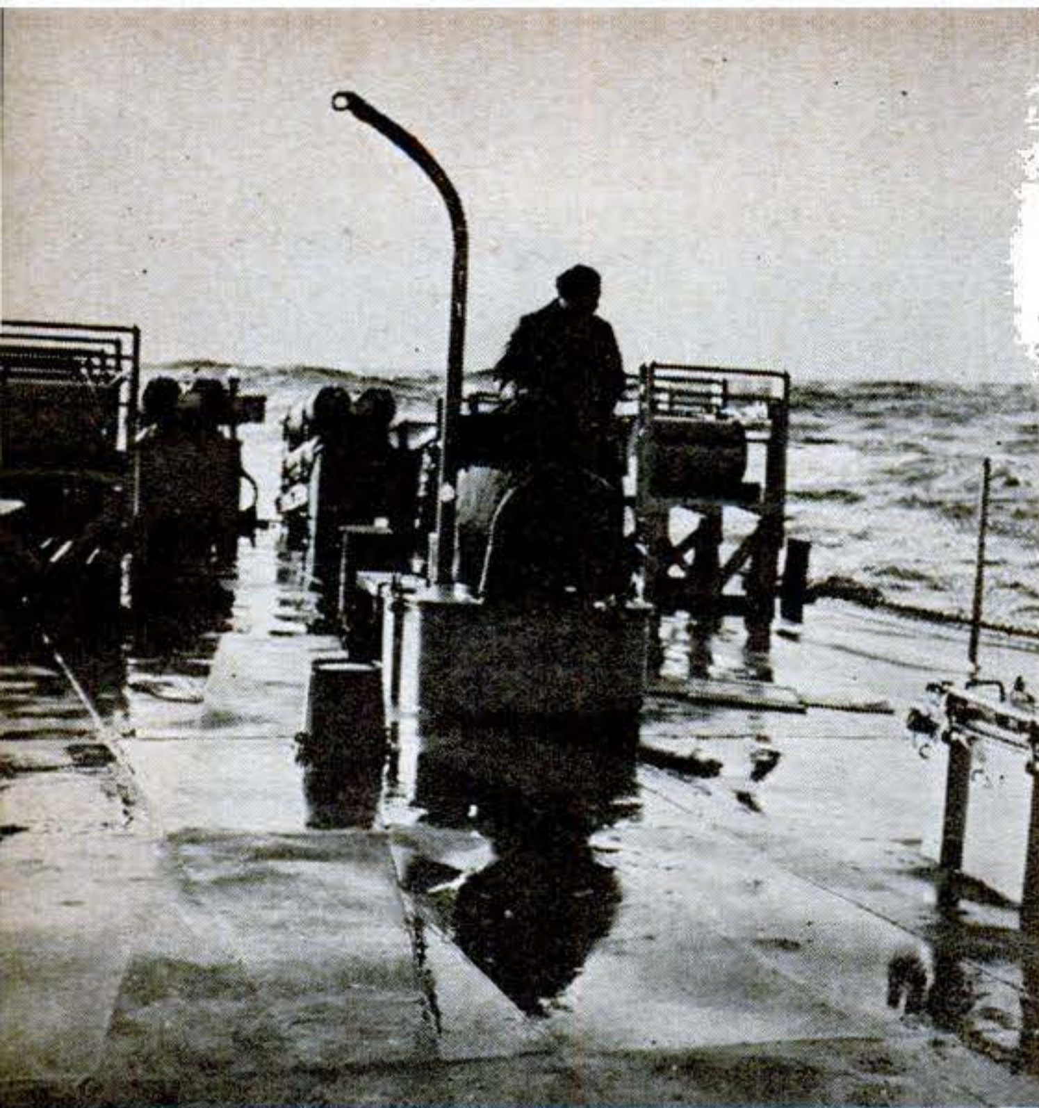
DEPTH CHARGES lie on sloping racks on the fantail, ready to be dropped astern as the DE races over the spot where a submarine has been detected. "Ashcans" are dropped in patterns designed to make it almost impossible for the U-boat to escape all
