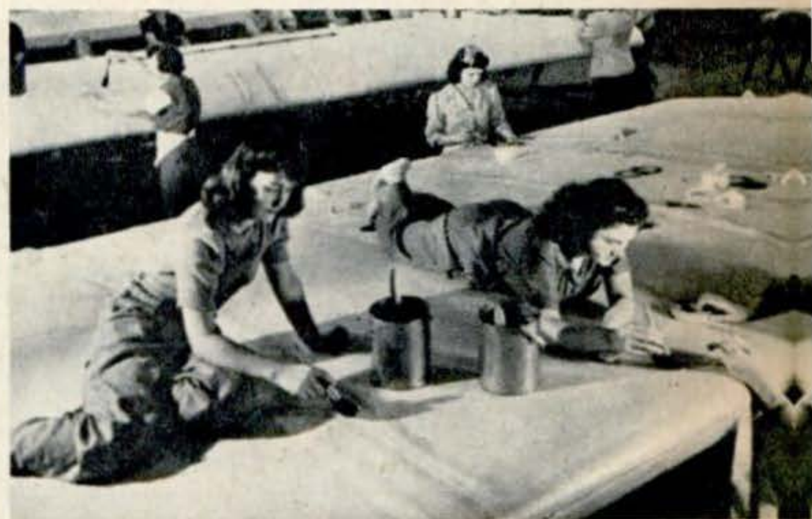
DOPING. Here two workers are covering stitches on a wing surface with tape and another is applying dope. Controlled temperature is necessary in doping
