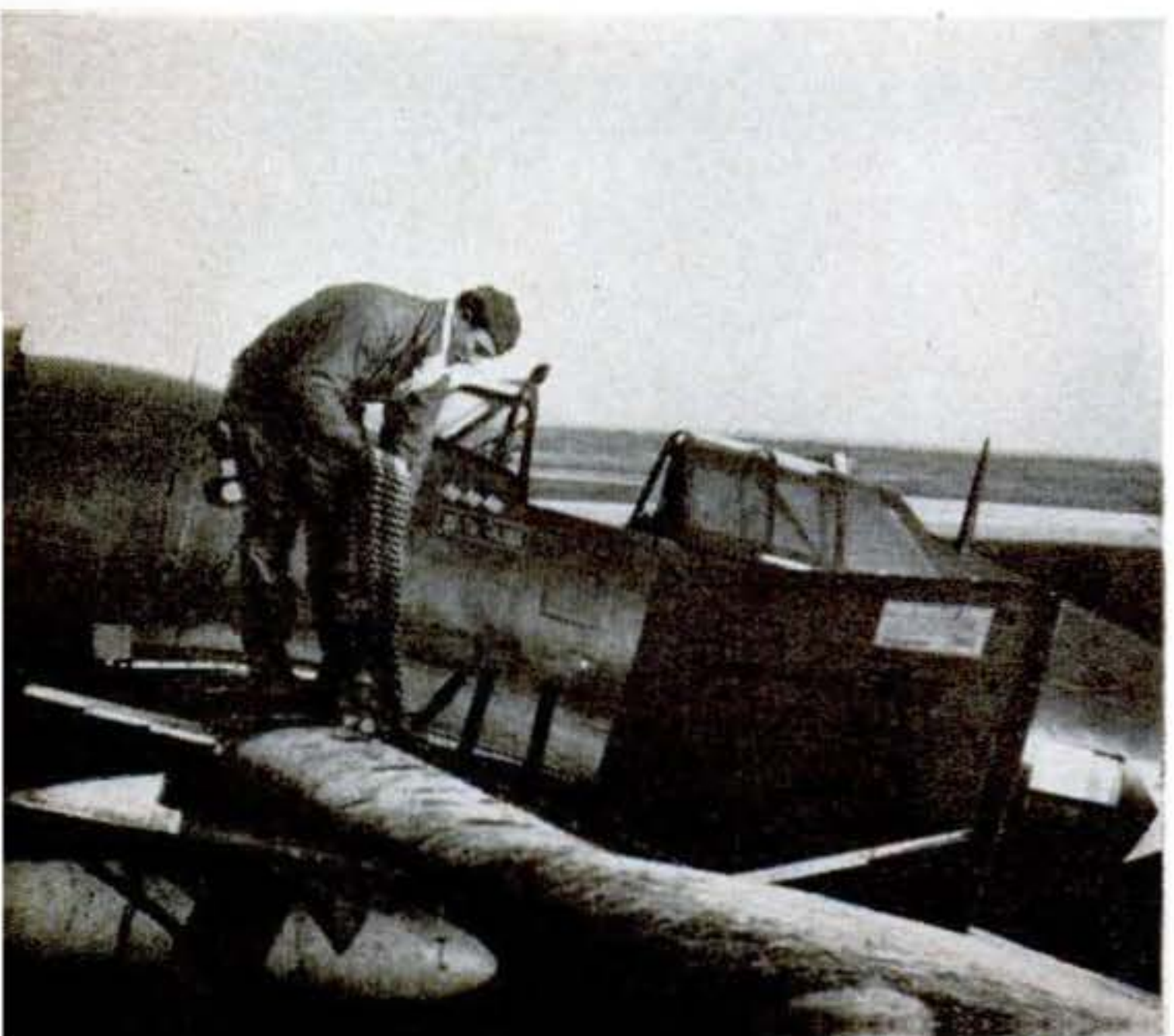
GUNS get a thorough going-over between missions. At left, below, one of the eight .50-calibers is being loaded through a hatch in the wing top. At regular intervals, the guns must be bore-sighted as a check on accuracy. A crane lifts the plane to flying position (right) so that targets can be lined up by eye through the barrels
