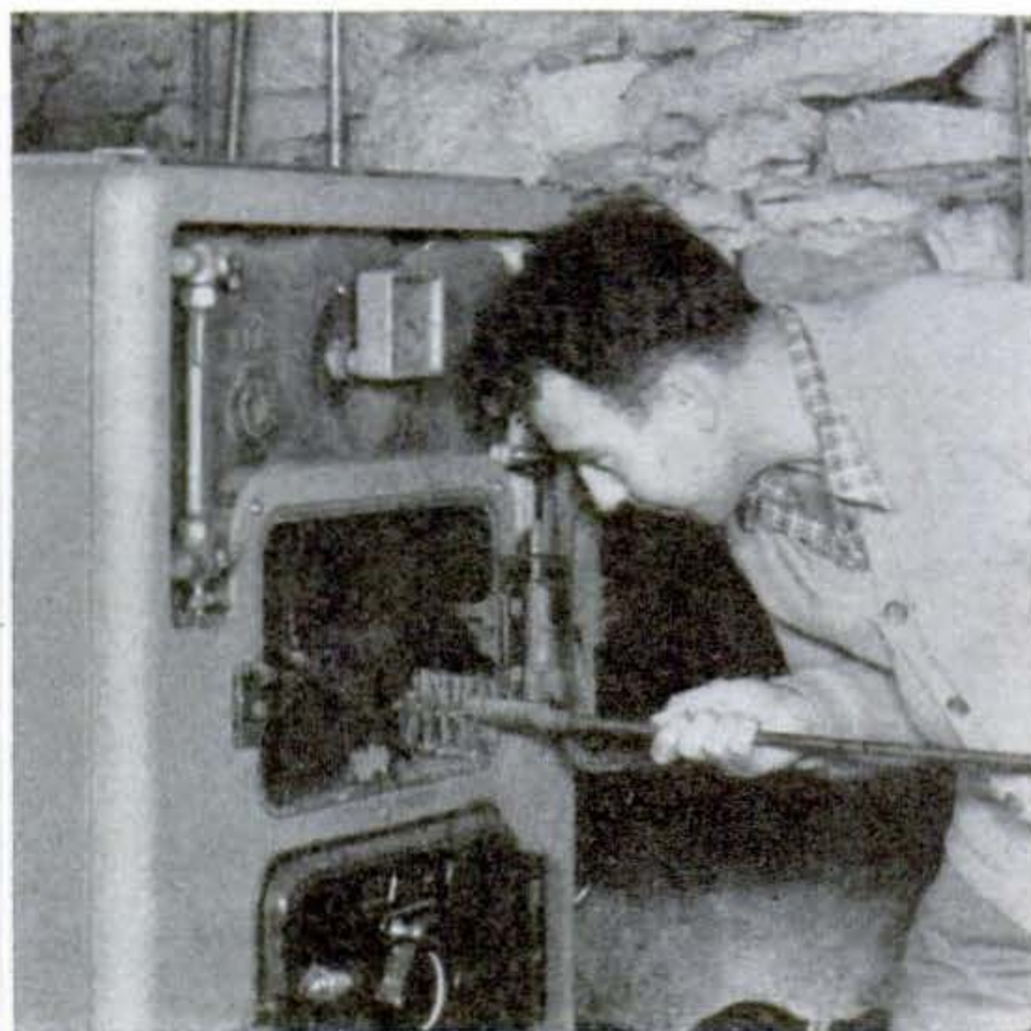
FLUE PASSAGES are cleaned with a wire brush to remove soot and scale that cut down heat
