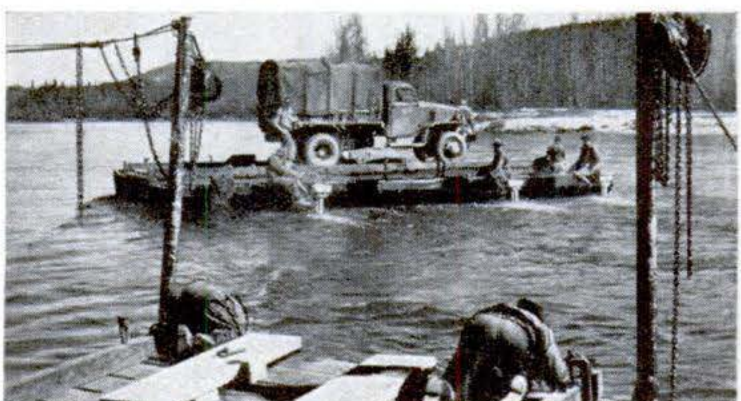
2 Ferries built quickly — here's how the Engineers do it! Several pontoons are decked together with standard bridge material and, with motors mounted, the ferry is ready!. Here 3 Evinrudes do a "triple screw" job pushing a truck up stream.
