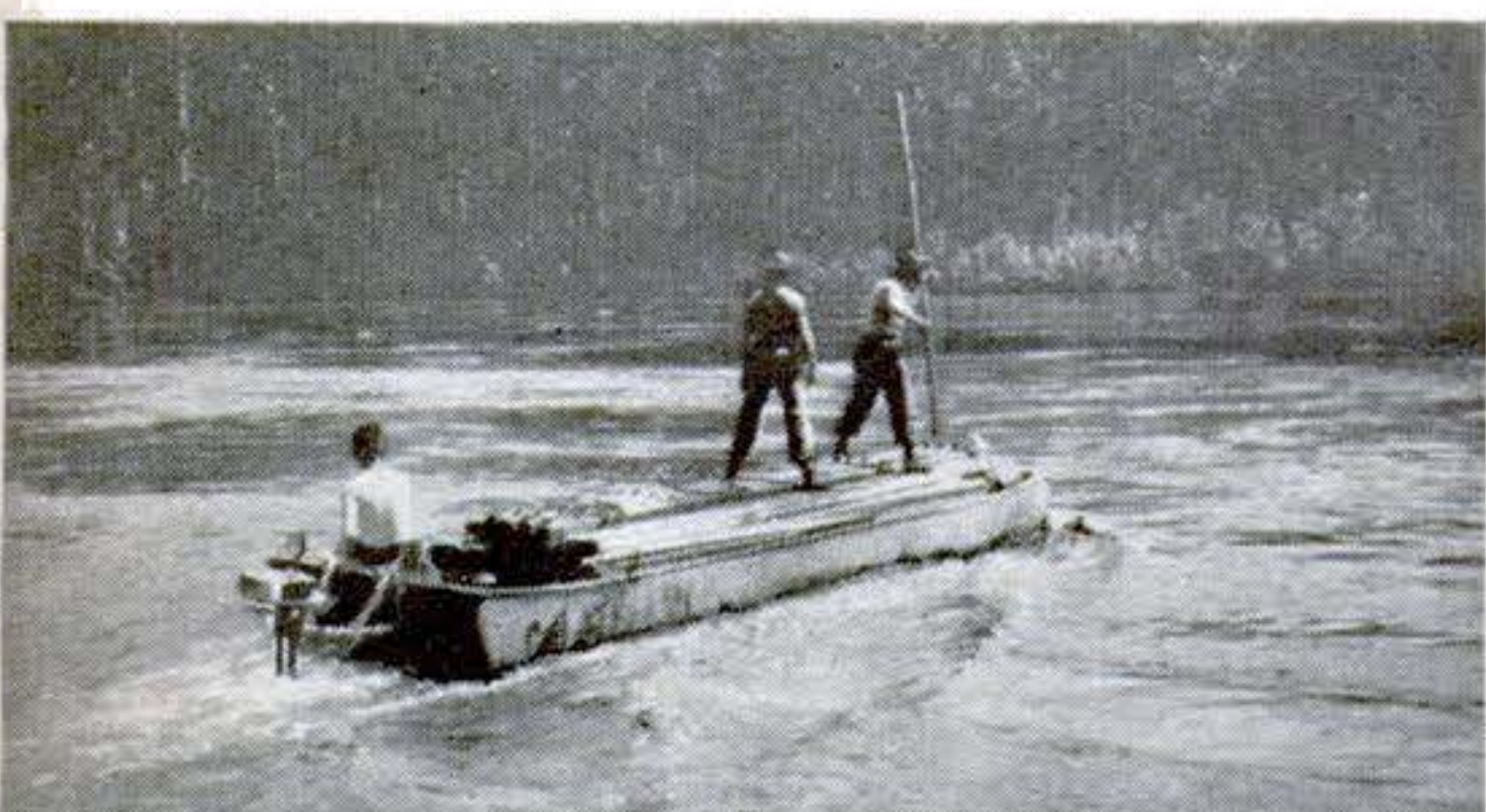
1 Mounted on the stern of a standard Engineers' ponton, (the Army term is ponton , not "pontoon"), this Evinrude makes fast work of transporting bridge material. It takes stamina as well as power to deliver the goods in this kind of service!
