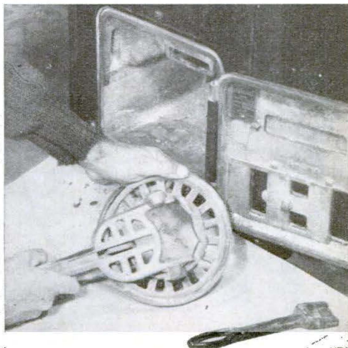
Grates require inspection for warping, cracks, and burned-out sections. A welding job will repair a clean break if the metal has not been burned away
