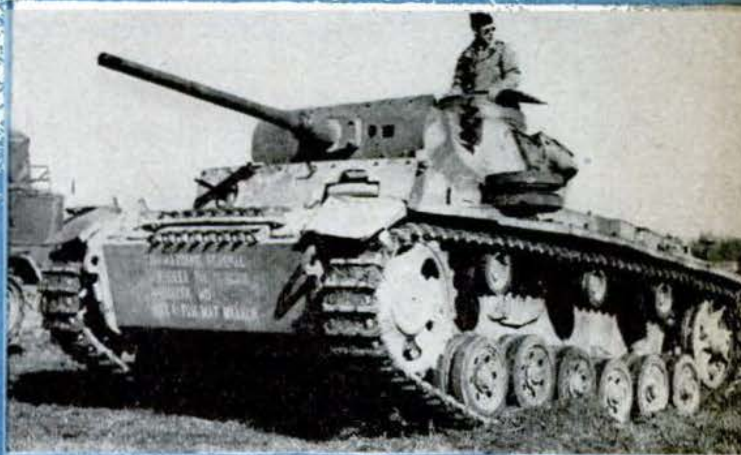
GERMAN MARK III TANK , which carries a 50-mm. cannon. Like the rocket gun, it was captured in North Africa. Much slower than American tanks, it is similar in characteristics to its big brother, the Mark IV, which is four tons heavier, carries thicker armor, and packs a big wallop with a 75-mm.
