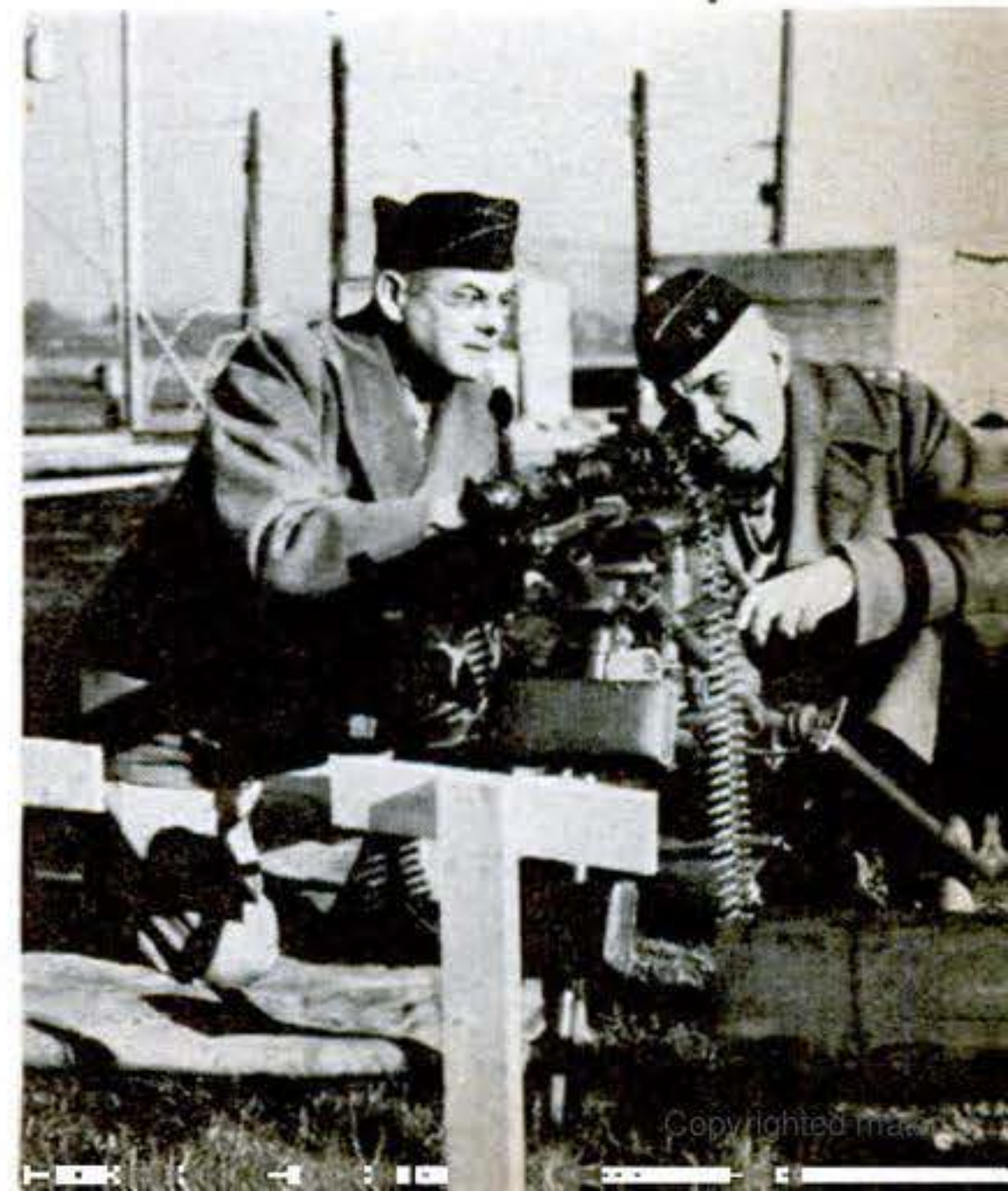
JAPANESE LIGHT MACHINE GUN, 6.5-mm., type 96 (1936). It is gas operated, magazine fed, air cooled; has bayonet for in-fighting
