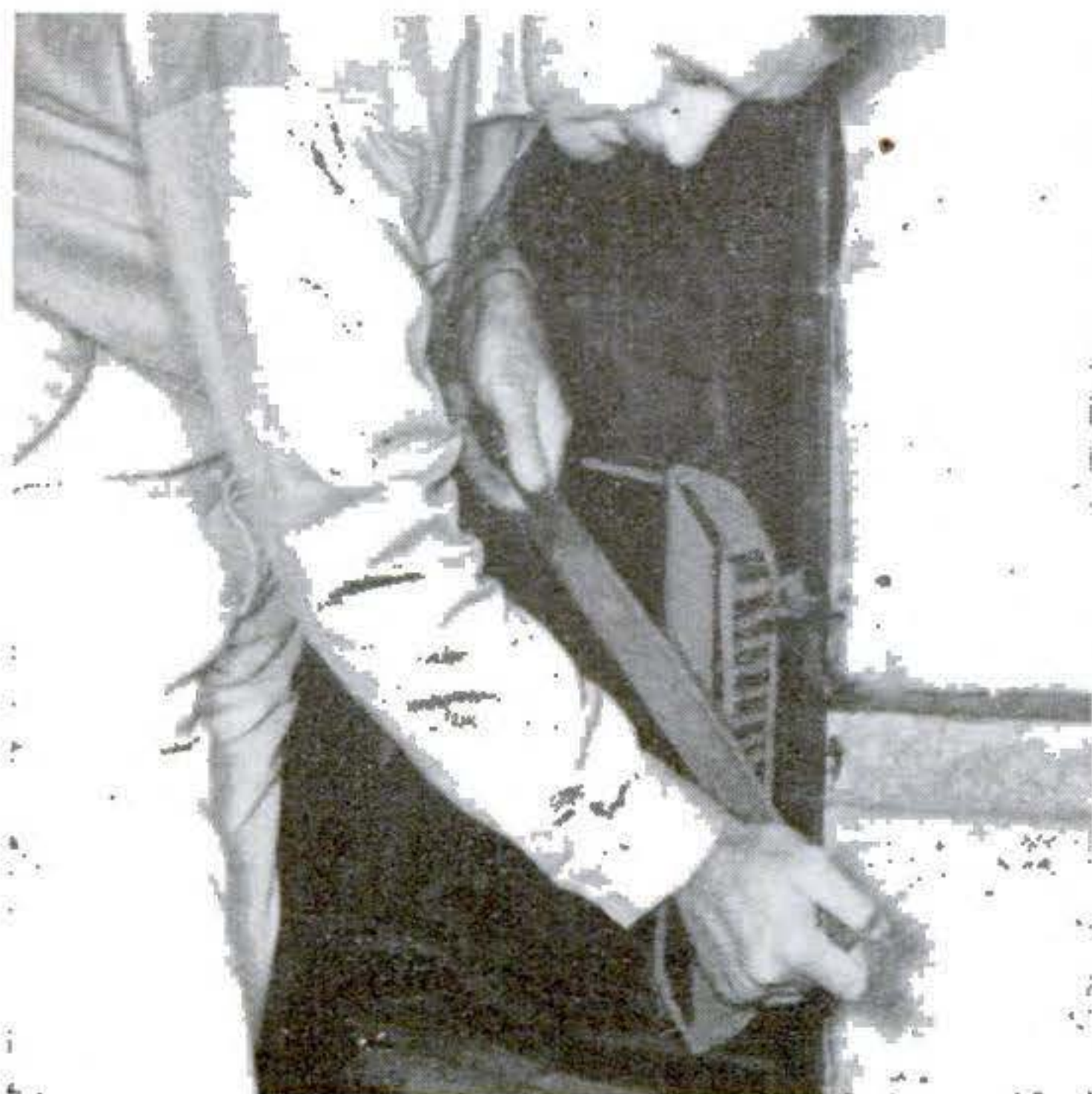
Warped doors should be cleaned, scraped, and filed on the high spots until they fit flat; otherwise they let in air, spoiling your control of the fire
