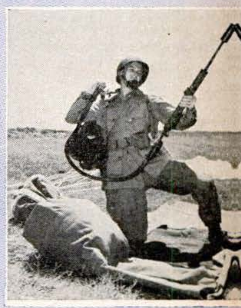
The paratrooper throws the harness over his shoulder. This projector, known as the M-1A1, can discharge a flame lasting 10 seconds
