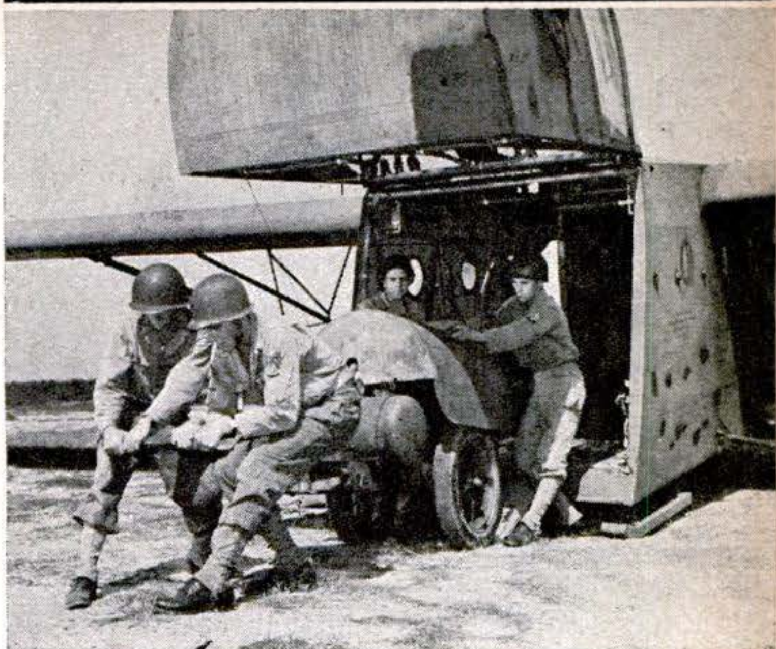
Out of a glider rolls the mobile, 1,200-pound power plant that speeds the work of the airborne engineers. It runs saws, drills, pumps. Tools may come in by glider or drop on 'chutes
