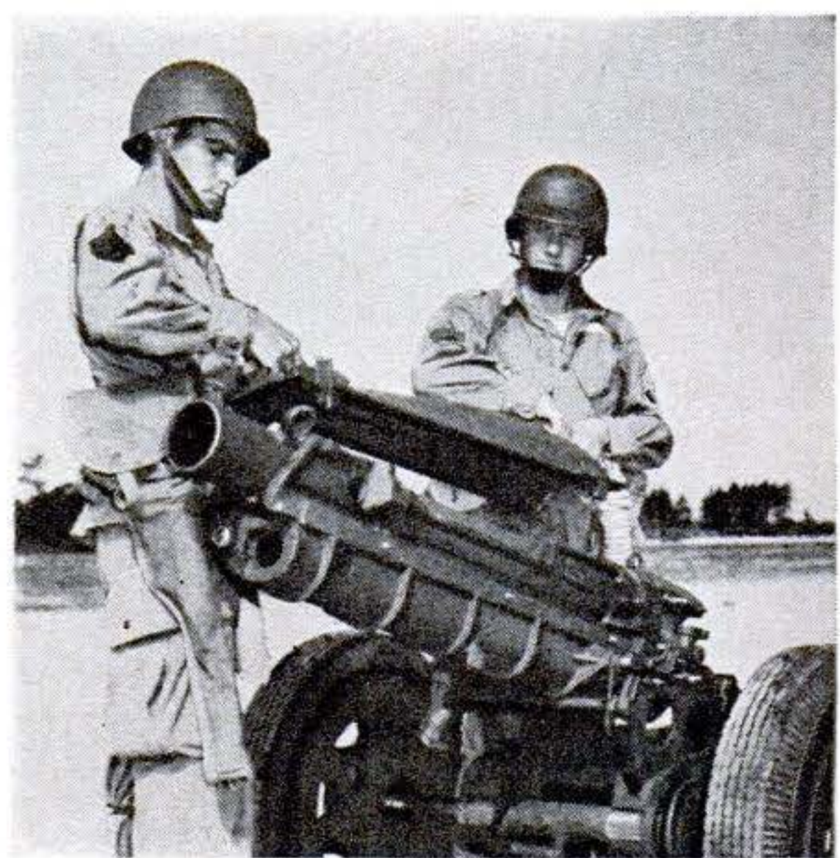
7 Within 6½ minutes, the 75-mm. field-piece is assembled and ready to fire. It is a regular mountain howitzer on a high-speed axle and rubber-tired wheels
